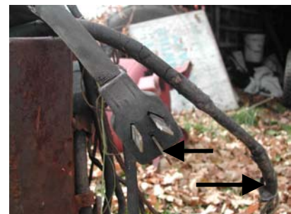
Figure 2-Ground prong loose and damaged insulation
