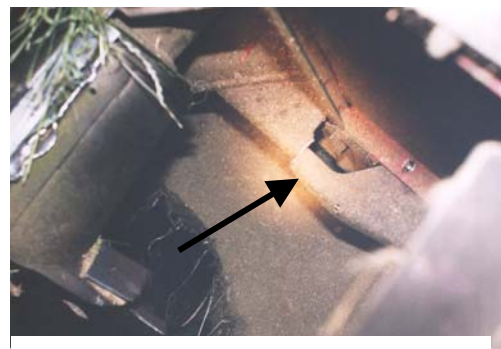
Figure 4 – Damaged Stone Guard
