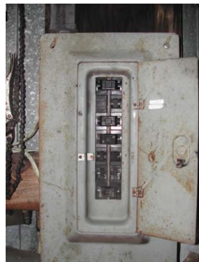
Figure 7. Unlabeled circuit breaker box in shed
