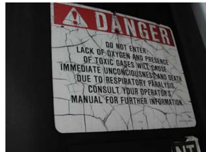
Photo 2. Silo Confined Space Warning Sign
