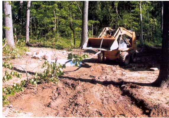
Figure 1. Skid-steer loader at scene
