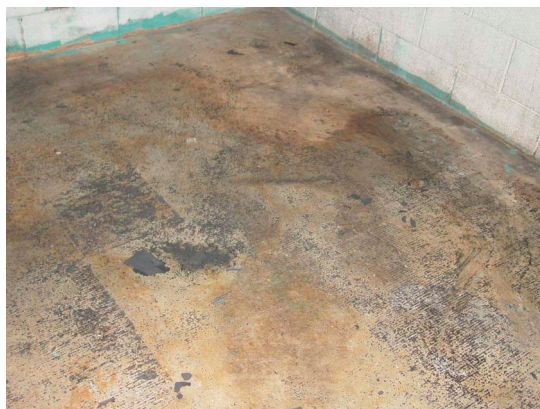
Figure 4. Carpet glue remnants on den concrete floor
