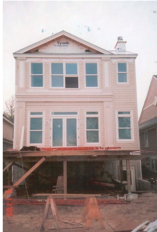
Figure 2. West Side of house
