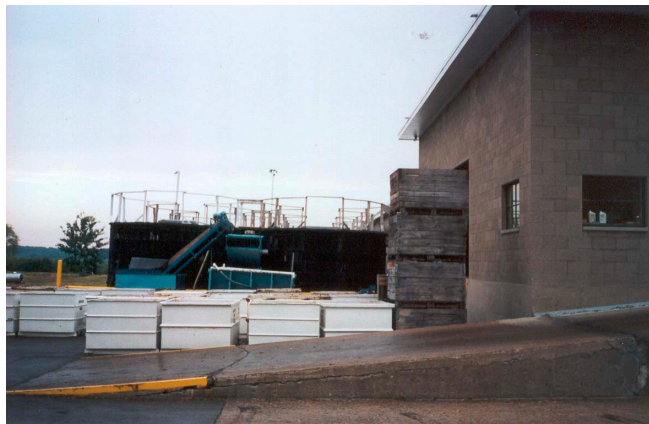
Figure 2. Loading station at primary tank room on day of incident
