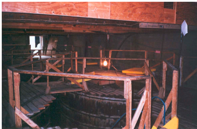
Figure 4. Inside of tank storage room-wood decking on and between tanks
