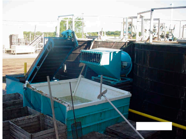
Figure 3. Loading station for primary tank room and location of deceased when supervising crew
