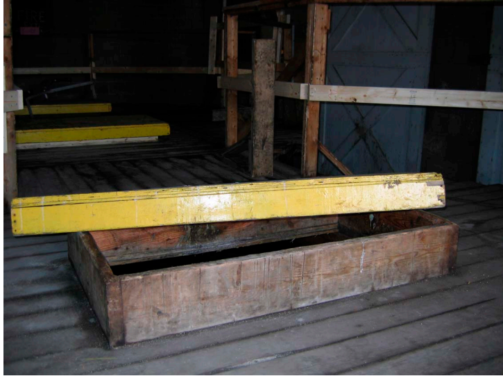
Figure 5. Example of tank opening and wood cover
