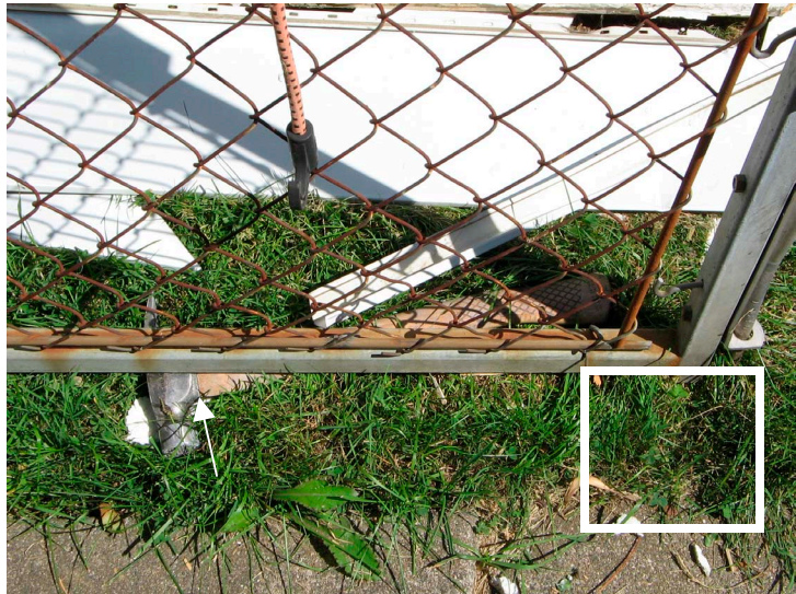
Figure 3. Hammer used to remove siding
