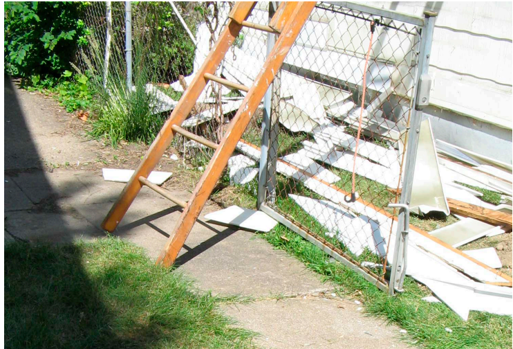
Figure 2. Ladder without safety feet on driveway against fence/gate
