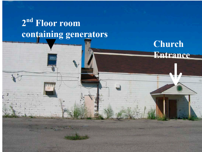
Figure 1. Incident scene showing outside of building
