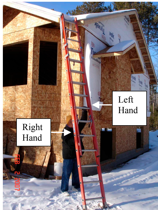
Figure 3. Re-enactment of the position of the coworker under ladder
