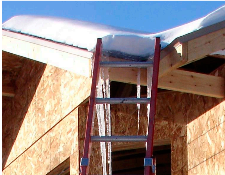
Figure 3. Ladder placed diagonally across inside corner
