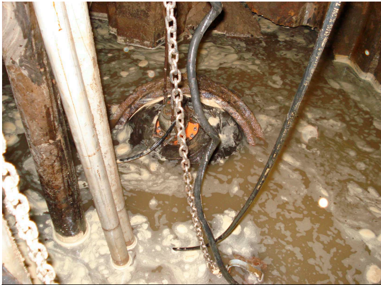
Figure 1. Pipe plug in broken sewer pipe at base of lift station
