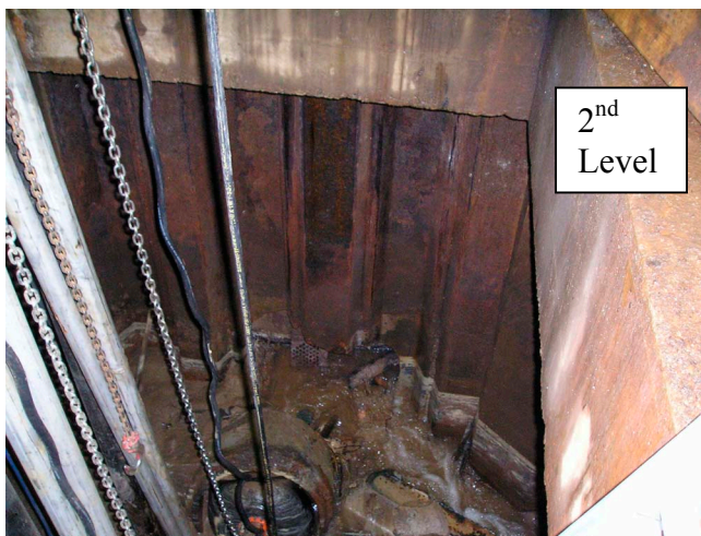
Figure 4. Pipe and plug at base of manhole after water was pumped
