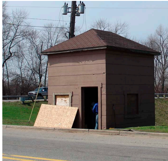
Figure 2. Lift station building
