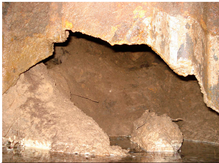
Figure 3. Manhole wall at location of pipe explosion
