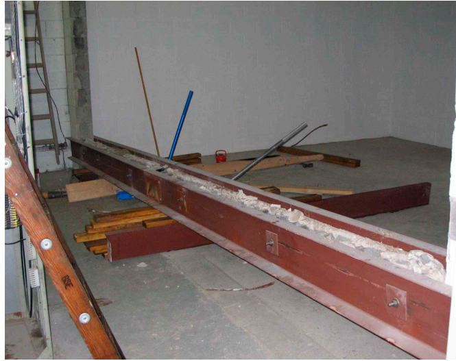
Figure 1. Header beam that fell onto decedent and two jacks used to raise beam from decedent.
