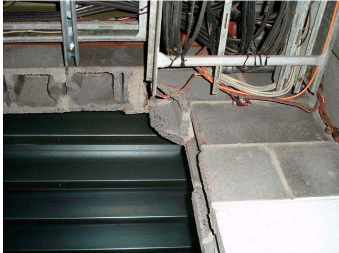
Figure 2. Location of cable tray interfering with original placement of C10 channels. Also shown is location of beam breakaway from the block wall.
