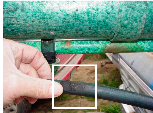
Figure 12. Burn mark on hose
