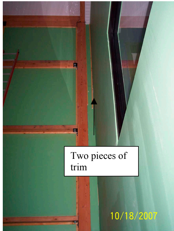
Figure 3. Placement of trim on west wall.
