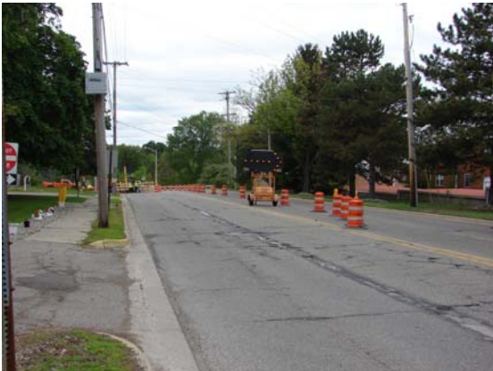
Figure 3. Looking west towards excavation site from south side of eastbound lanes of 4-lane roadway
