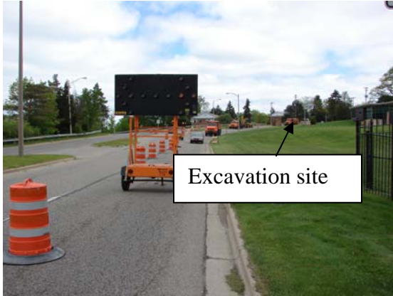
Figure 2. Incident roadway looking northeast at lane taper
