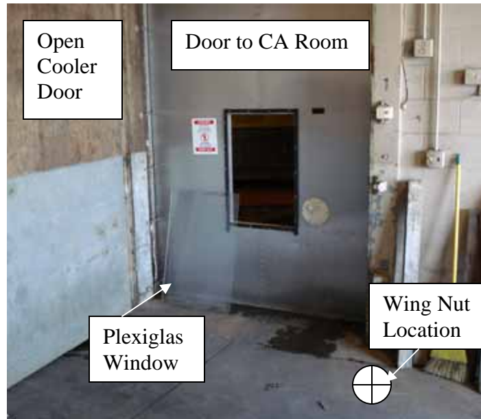
Figure 1. Outer door, inner aluminum door, Plexiglas window, opening to CA room, warning sign, wing nuts location
