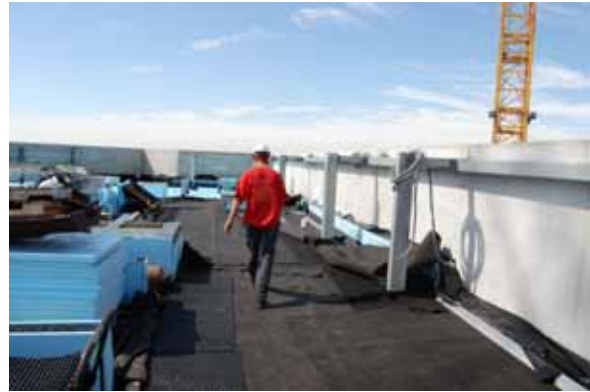
Figure 2. Position of tower crane in relation to roof area
