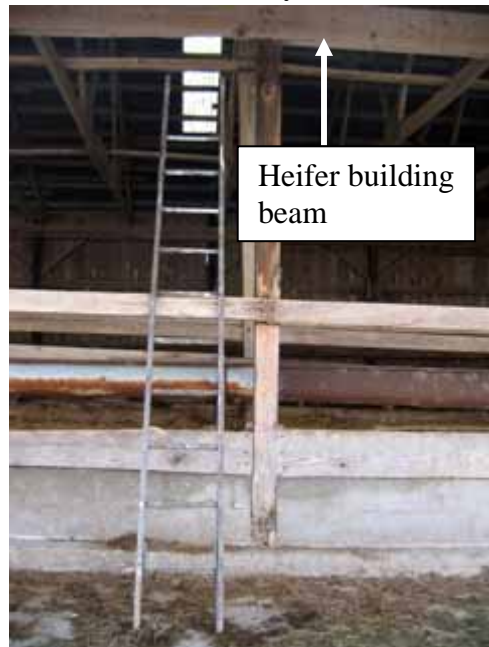
Figure 4. Ladder placed under (not supported) by the building beam and against fence railing
