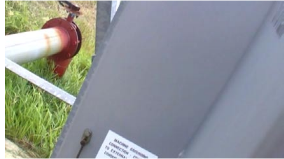
Figure 4. Machine ground of Reinke central pivot.
