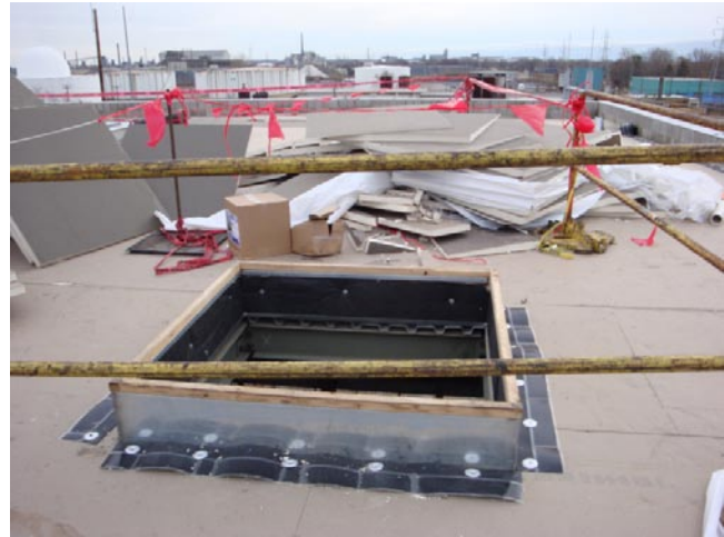
Figure 1. Roof hatch involved in incident. Note nearby pile of insulation sheets.
