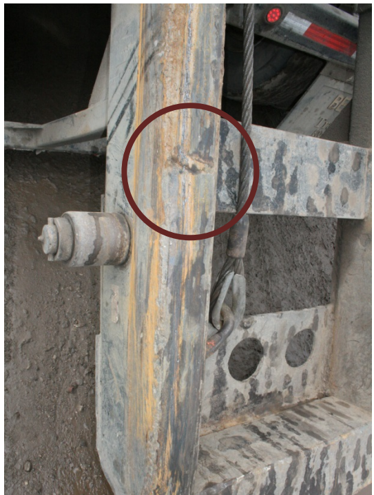
Figure 5. Fresh gouge mark on the driver's side trailer bed rail.
