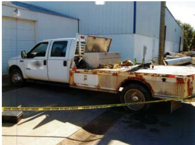
Figure 2. Truck involved in incident. Truck facing east, front wheels in trench
