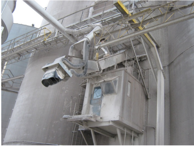
Figure 6. Looking up at the load out room and lowered steps.
