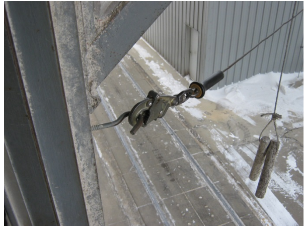
Figure 8. DBI Sala-Ultra Lok RSQ Self-Retracting Lifeline (SRL) attached to load out room.
