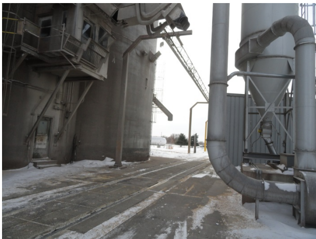
Figure 5. Overview of incident scene. Steps to railcar in retracted position.
