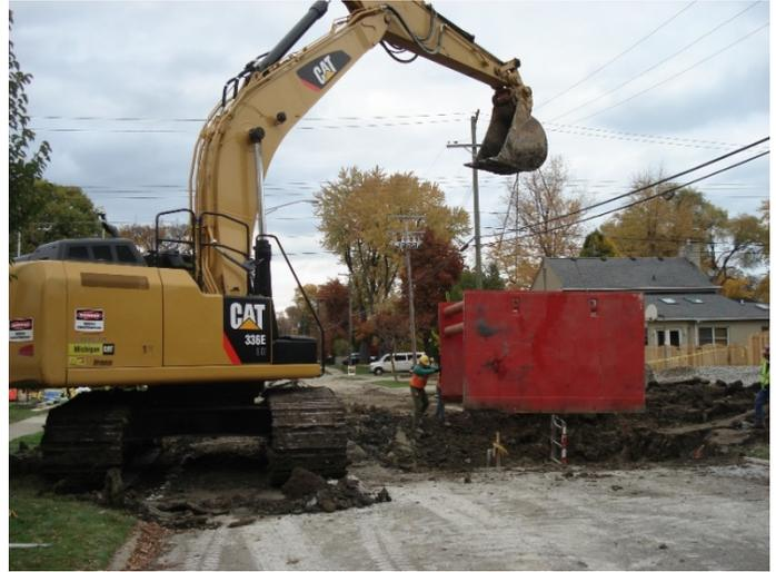
*Figure 2. Placement of trench box after road removal*
