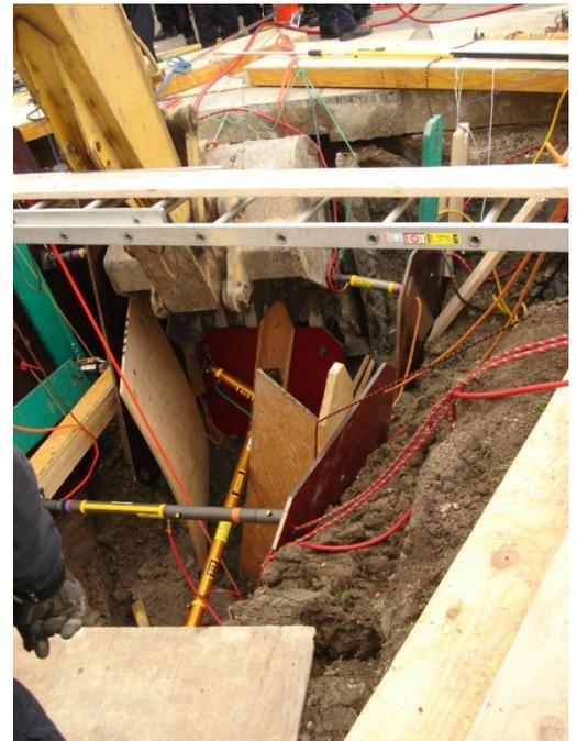
*Figure 1. Recovery operations trench wall support*
