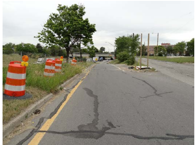
Photo 5. Construction materials at entrance ramp #2
