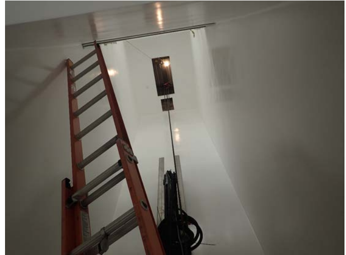
Photo 5. View of shaft way looking up from the ground floor.
