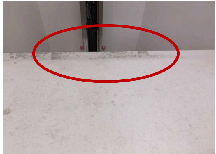
Photo 3. Ladder marks on edge of second floor
