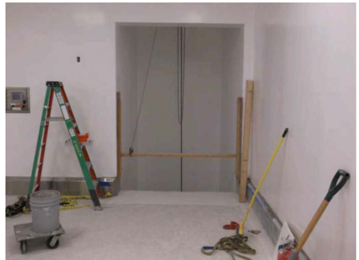
Photo 2. Lifeline attached to midrail at time of incident
