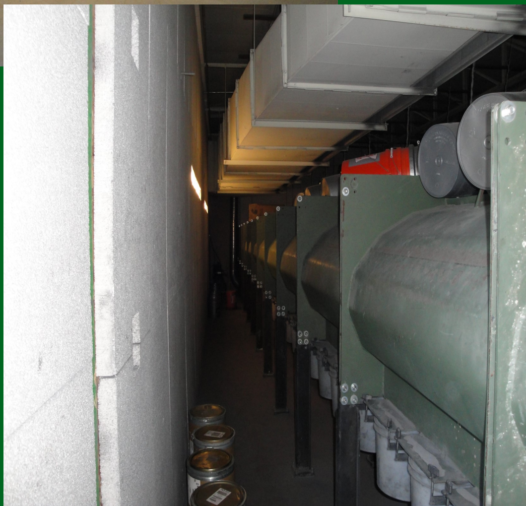
Picture 2 Range Trap behind 14 Computerized Firing Lanes
