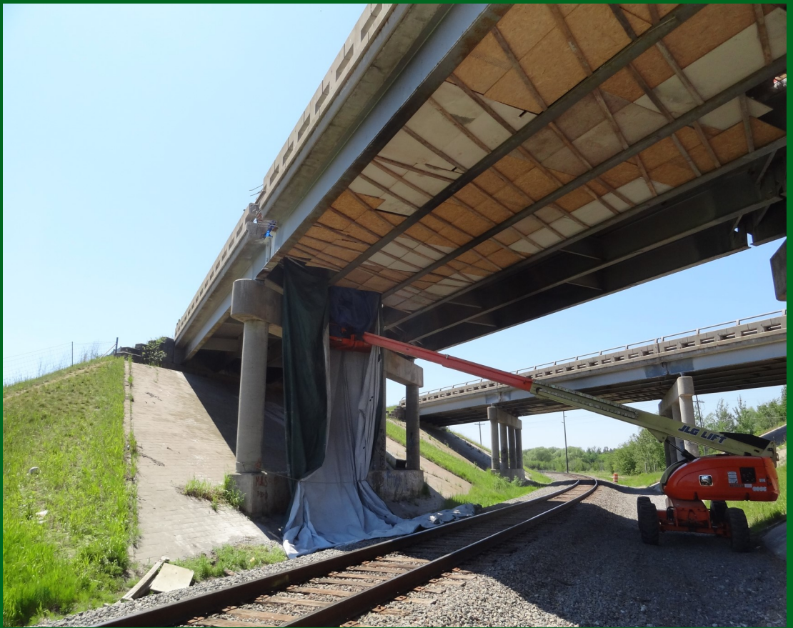
Picture 4 Abrasive Blasting of Structural Steel Coated with Lead- Containing Paint
