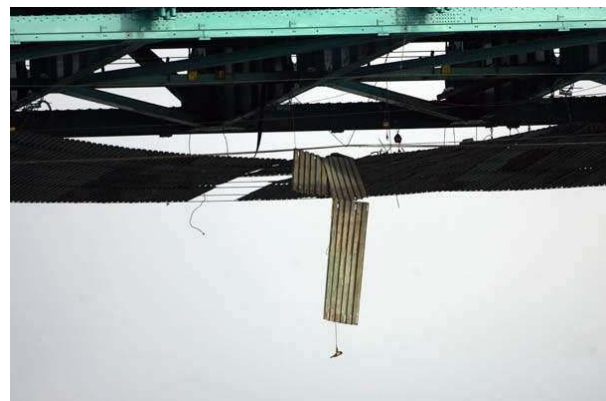
Case 2. Construction worker died when the cantenary suspended scaffold platform sheet collapsed
