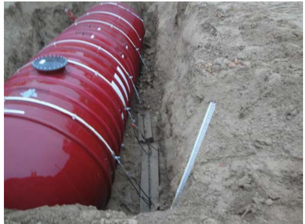
Case 113. Sprinkler fitter/pipefitter died when pinned against an excavation wall by a tank which moved due to the collapse of another of the excavation's walls
