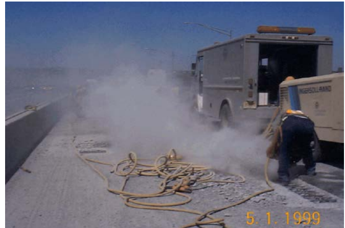
Example of respirable quartz-containing dust as a highway construction worker cuts cement.
