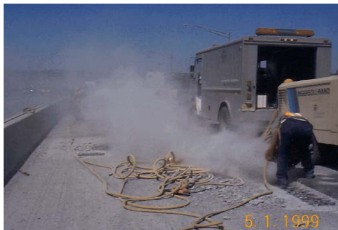
Example of respirable quartz-containing dust as a highway construction worker cuts cement.
