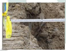
A male pipe layer in his 40s died in a trench wall collapse while installing drain tile pipe. The trench had a 1½-foot seam of wet sand at its base and then 5 feet of wet clay. Falling clay forced a shovel to strike his right side, pinning him against the opposite side of the excavation.
