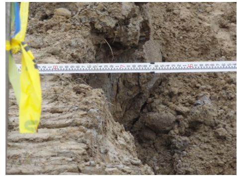
A male pipe layer in his 40s died in a trench wall collapse while installing drain tile pipe. The trench had a 1½-foot seam of wet sand at its base and then 5 feet of wet clay. Falling clay forced a shovel to strike his right side, pinning him against the opposite side of the excavation.
