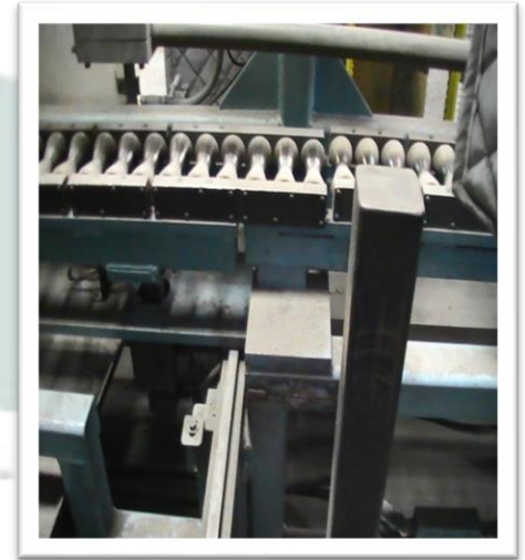
Lack of guards for pinch points is one of the causes of occupational crushing injuries
