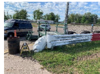
Pit exit area where the flagman was standing.
