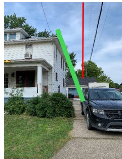
Incident scene: ladder placement (in green) and overhead line location (in red).
