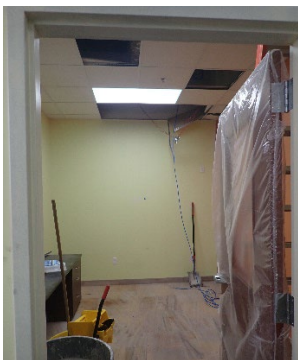
The room where the work was being performed.
