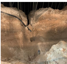
View of the trench after recovery.
