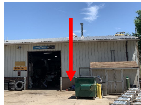
Location where the ladder was placed when the fall occurred.
