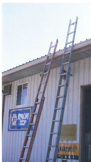
Ladders used at the job site. The laborer fell from the ladder on the right. The ladder is not in the location of the fall in this photo.
