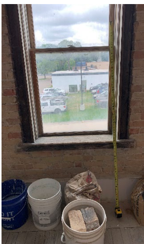
Window opening used to dispose of demolition debris.
