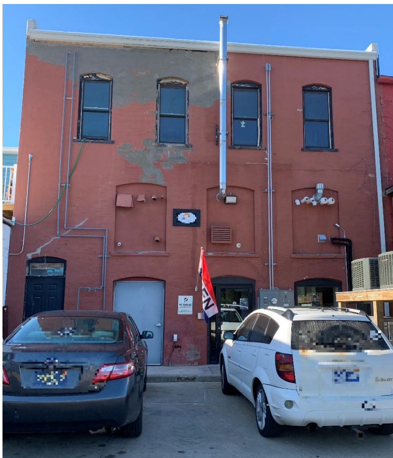
Ground level view up to second floor apartment.
