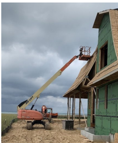
View of the construction project and the boom lift utilized to elevate the workers. Source: MIOSHA
