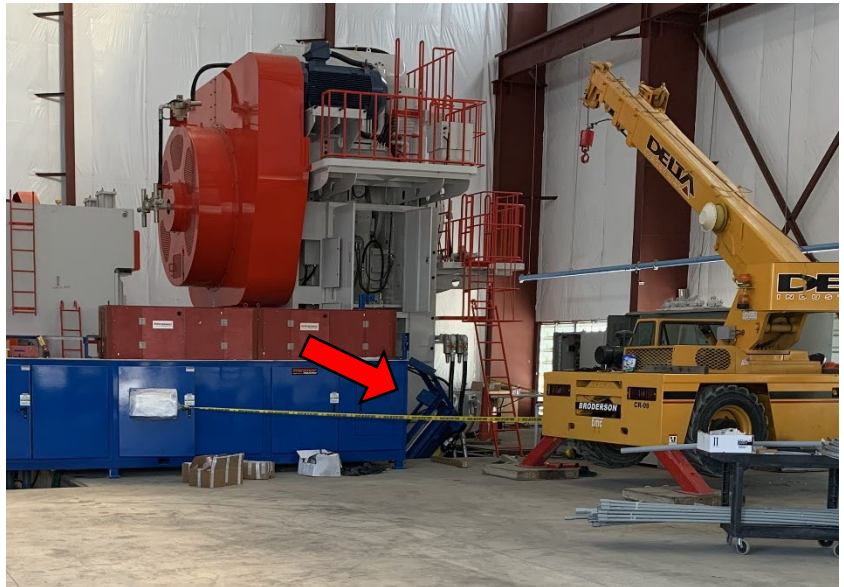
Wide view of the incident location. The crane is to the right, open pit under blue equipment, and motor assembly (red arrow).
