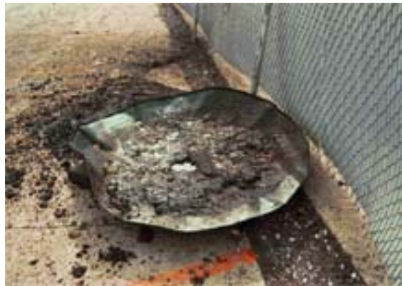
Tank Base Against Plant Fence
