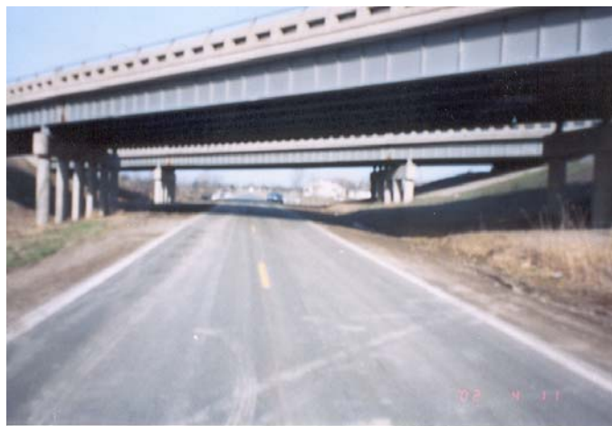
Figure 2. Road where incident took place
