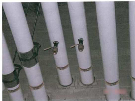
Figure 2 Closed Pressure Relief Valves
