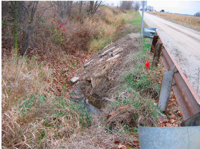
Figure 1. View of ditch from 2-track road. Looking to operator's left.
