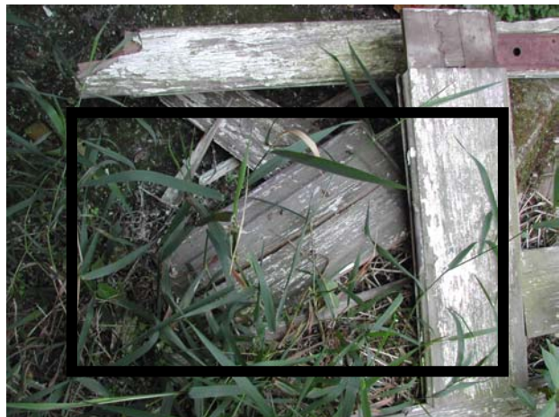
Figure 6. Cracked doorframe
