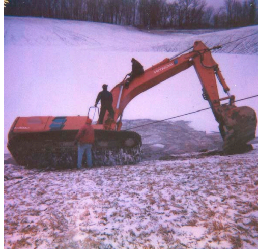
Figure 4. Divers hooking cables to excavator
