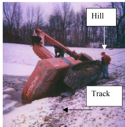
Figure 2. Excavator tracking along water edge toward wall to ascend
