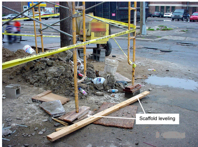
Figure 2. Example of scaffold leveling
