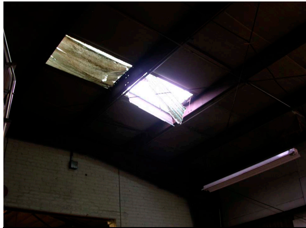
Photo 1. Picture of broken skylight
