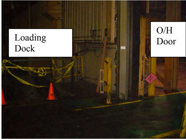
Figure 4. Position of loading dock in relation to overhead (O/H) door
