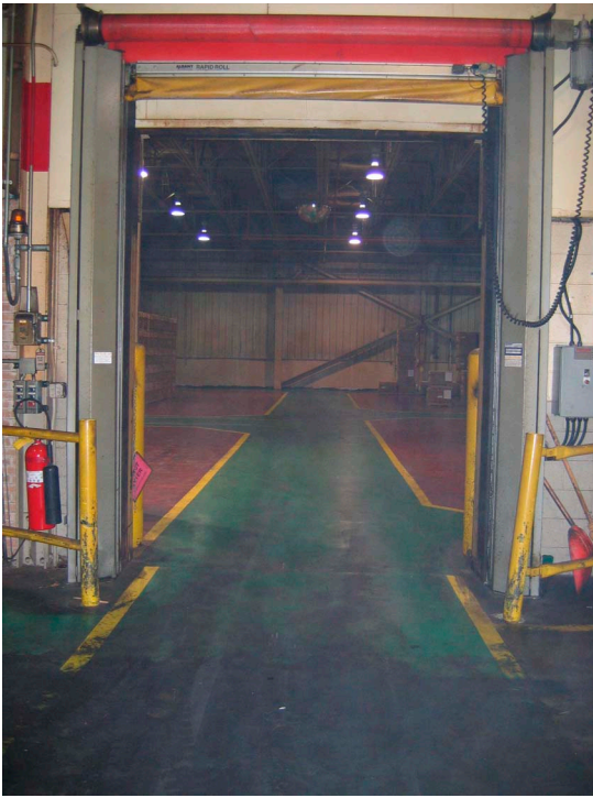
Figure 3. Overhead door near loading dock platform
