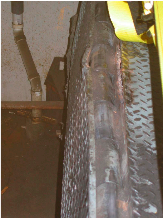
Figure 5. Bent dock boarding plate
