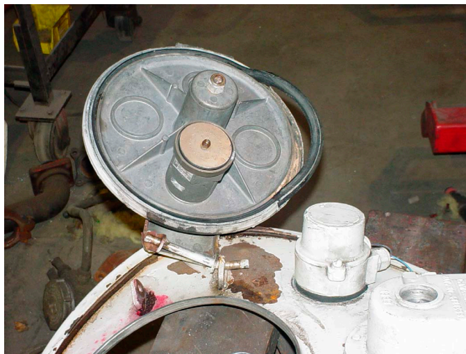
Figure 5. Condition of Compartment #4 10-inch lid after the explosion
